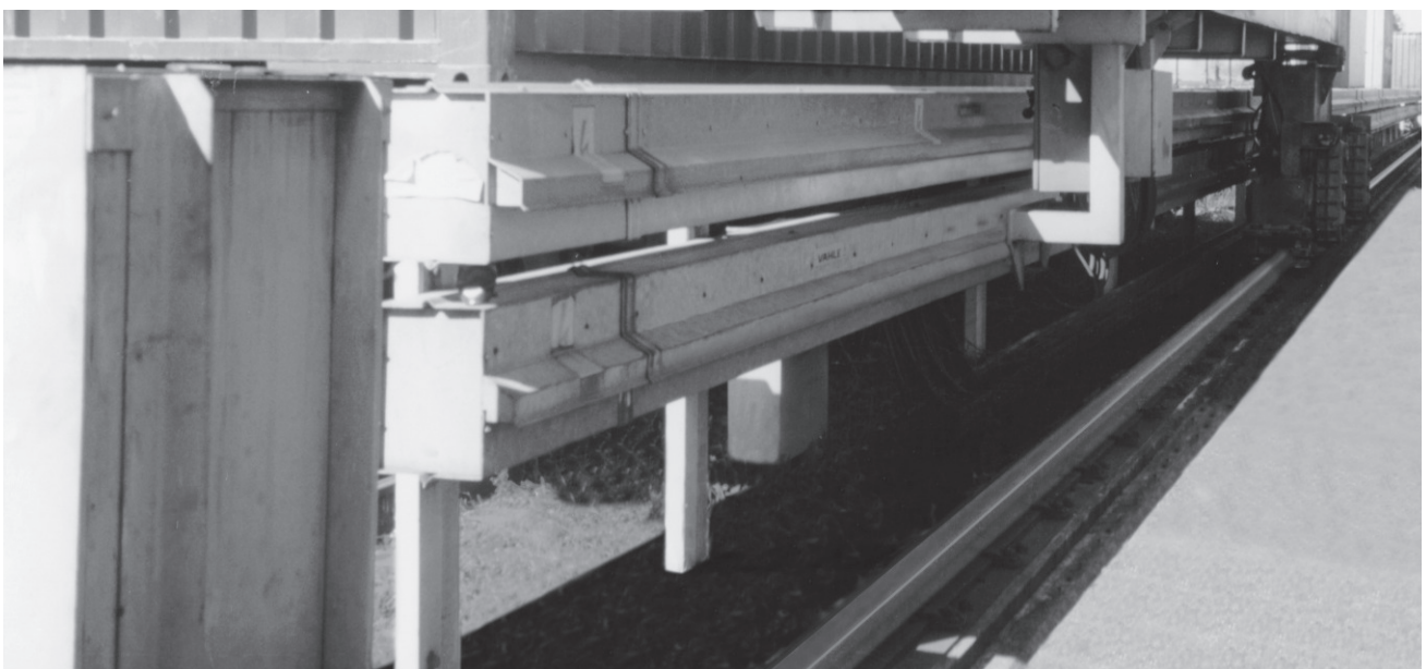
VAHLE FK-system for container terminal
