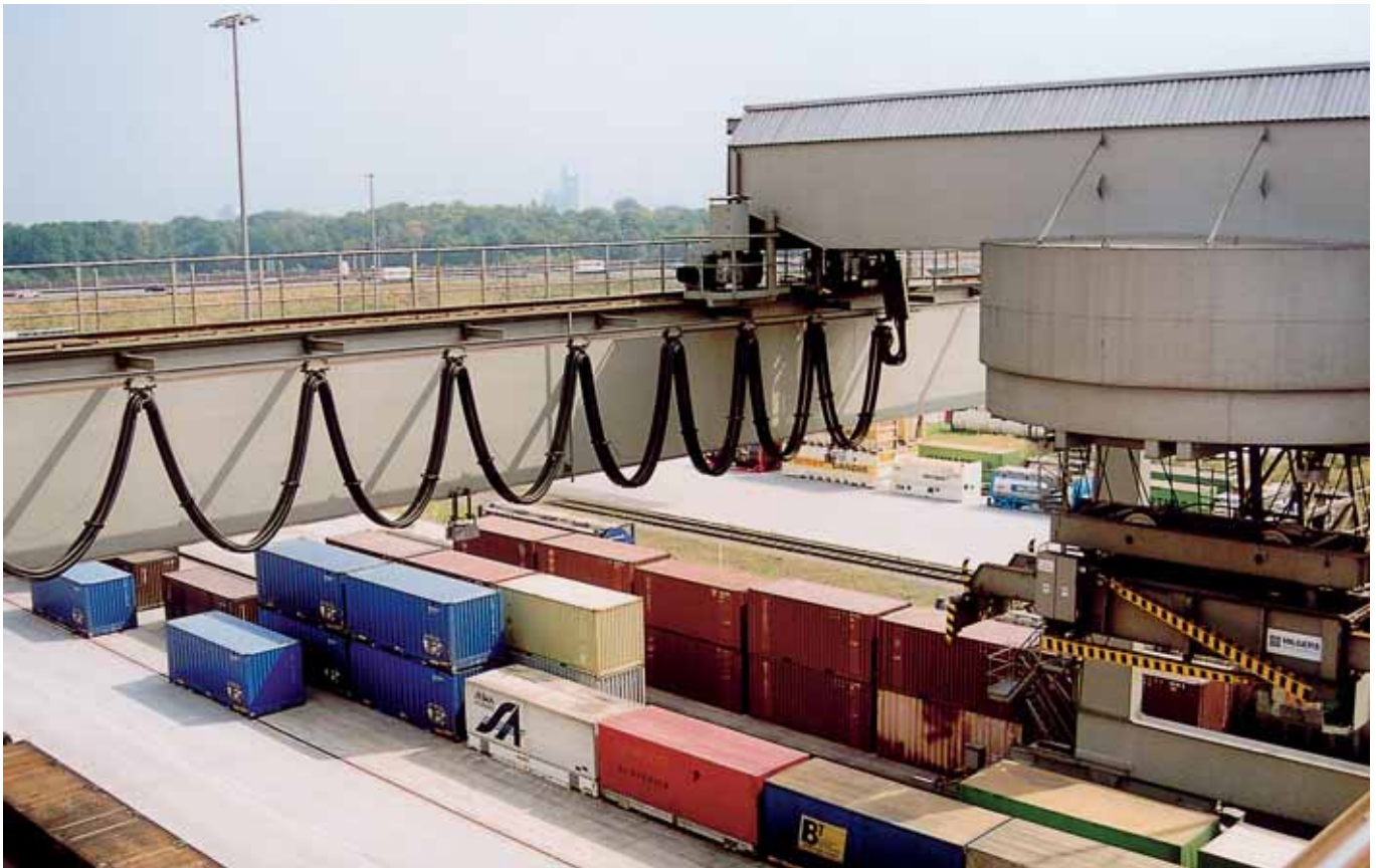
Cable carrier at a container crane
